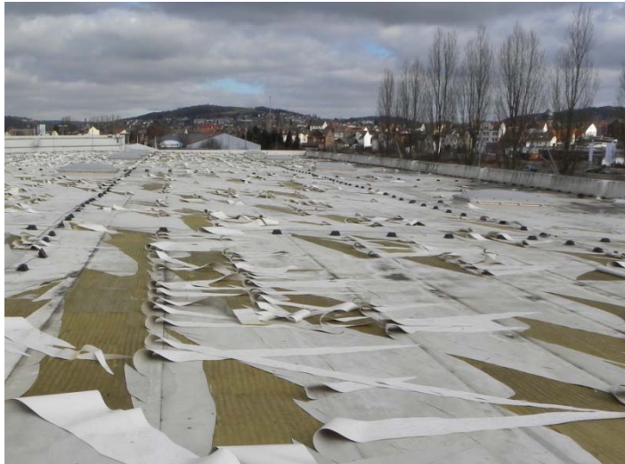
Examples of two improper unreinforced membranes from the past
