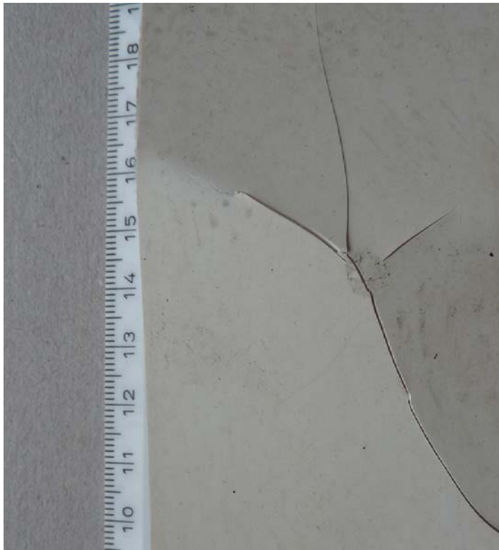
Shatter crack after determination of resistance to impact (acc. DIN EN 12 691 on -10°C (2 years aged membrane, EVA/PVC, 1,5 mm).
