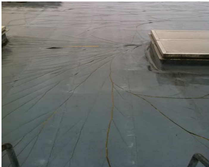
Examples of two improper unreinforced membranes from the past
